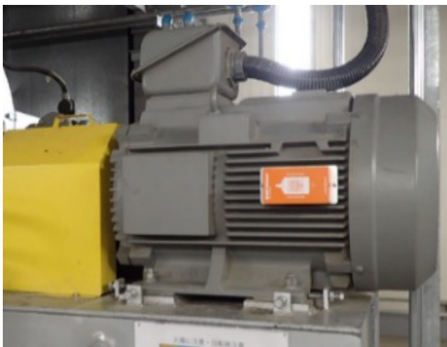
Deployed SMS Sensor Device on the IDF Motor
