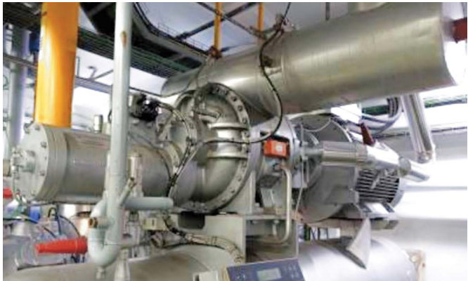
Figure 7. OtoSense SMS sensor installed on a customer facility compressor.
