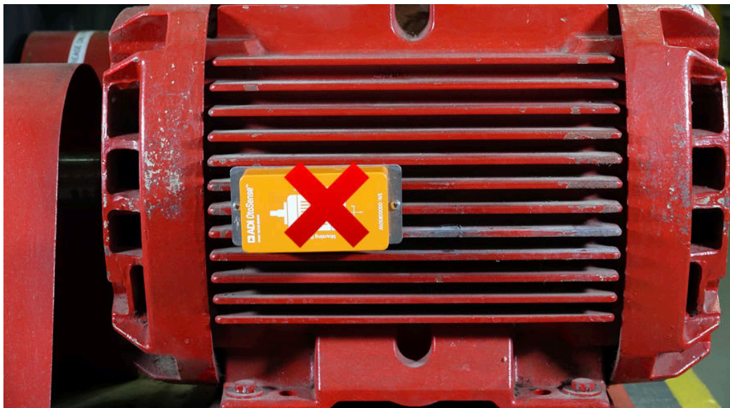
Figure 34. Incorrect Positioning – an SMS device installed in the front area relative to the motor shaft
