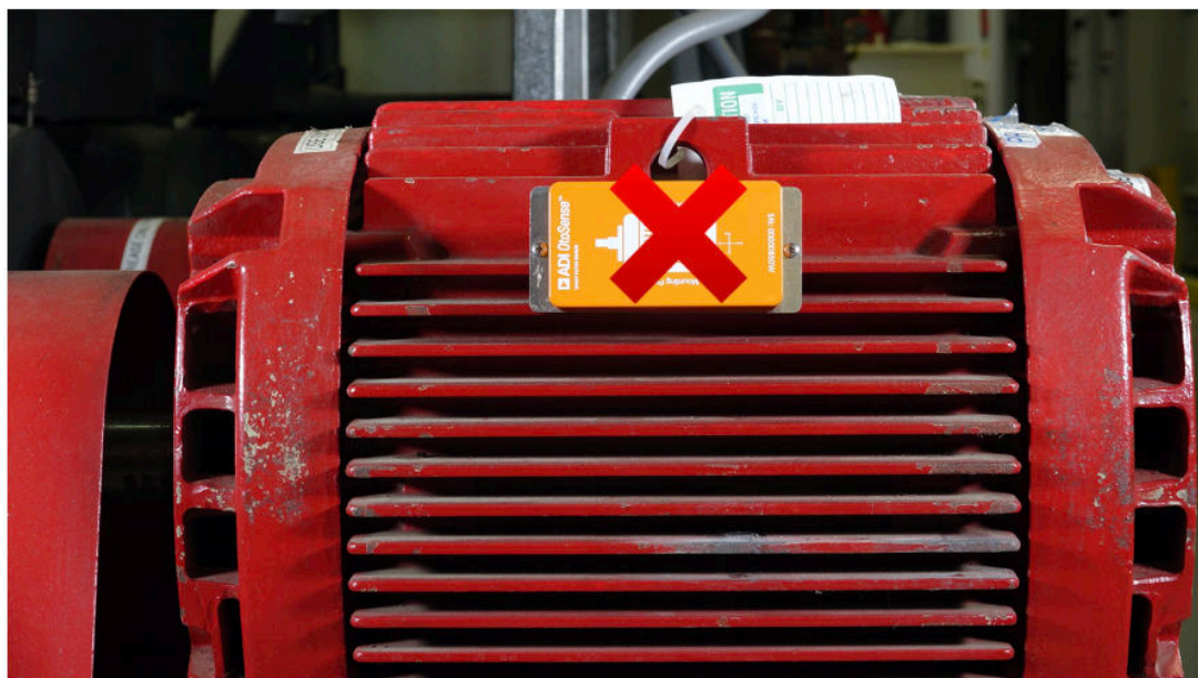
Figure 33. Incorrect Positioning – An SMS device installed at the top of the motor
