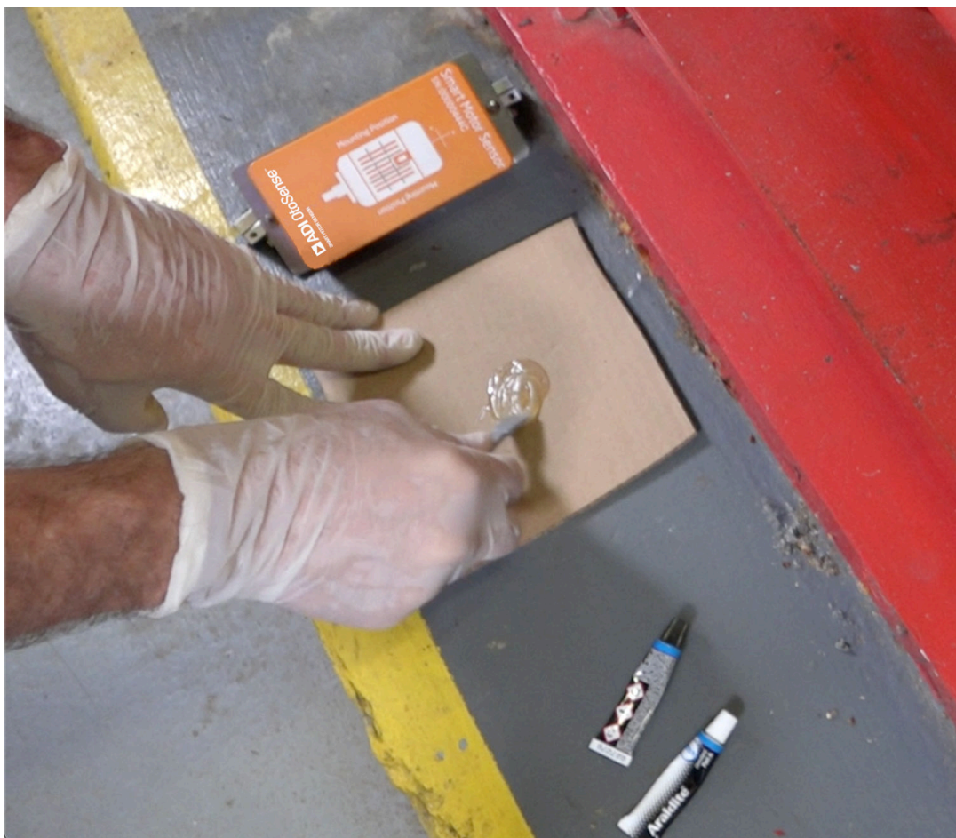
Figure 41. Mixing the bi-component adhesive
